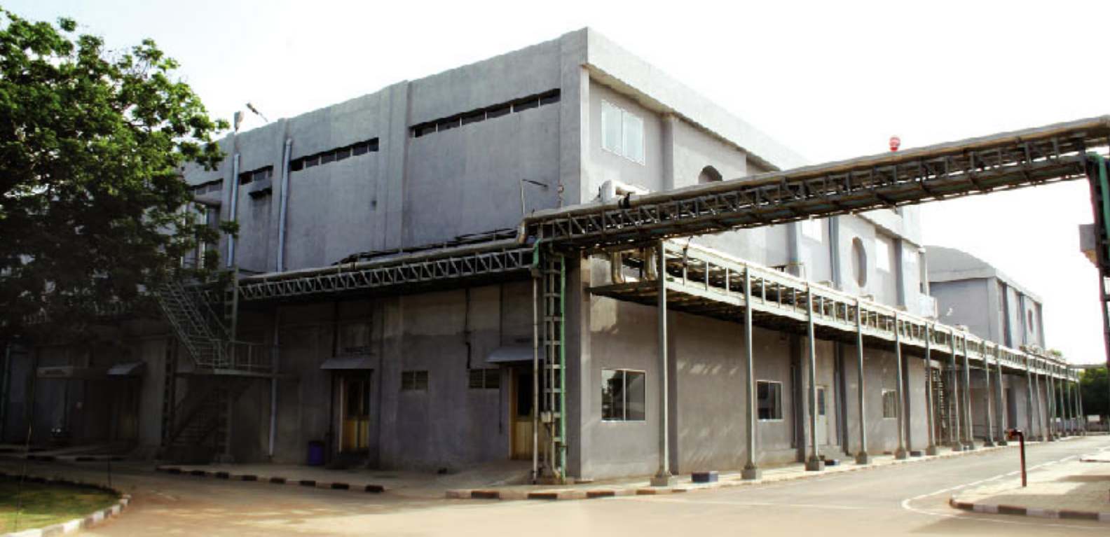
Active Pharmaceutical Ingredient (API) manufacturing facility at Indrad, Gujarat
