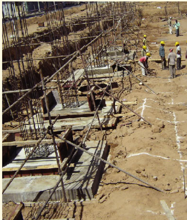
Site for new sterile manufacturing facility at Indrad, Gujarat
