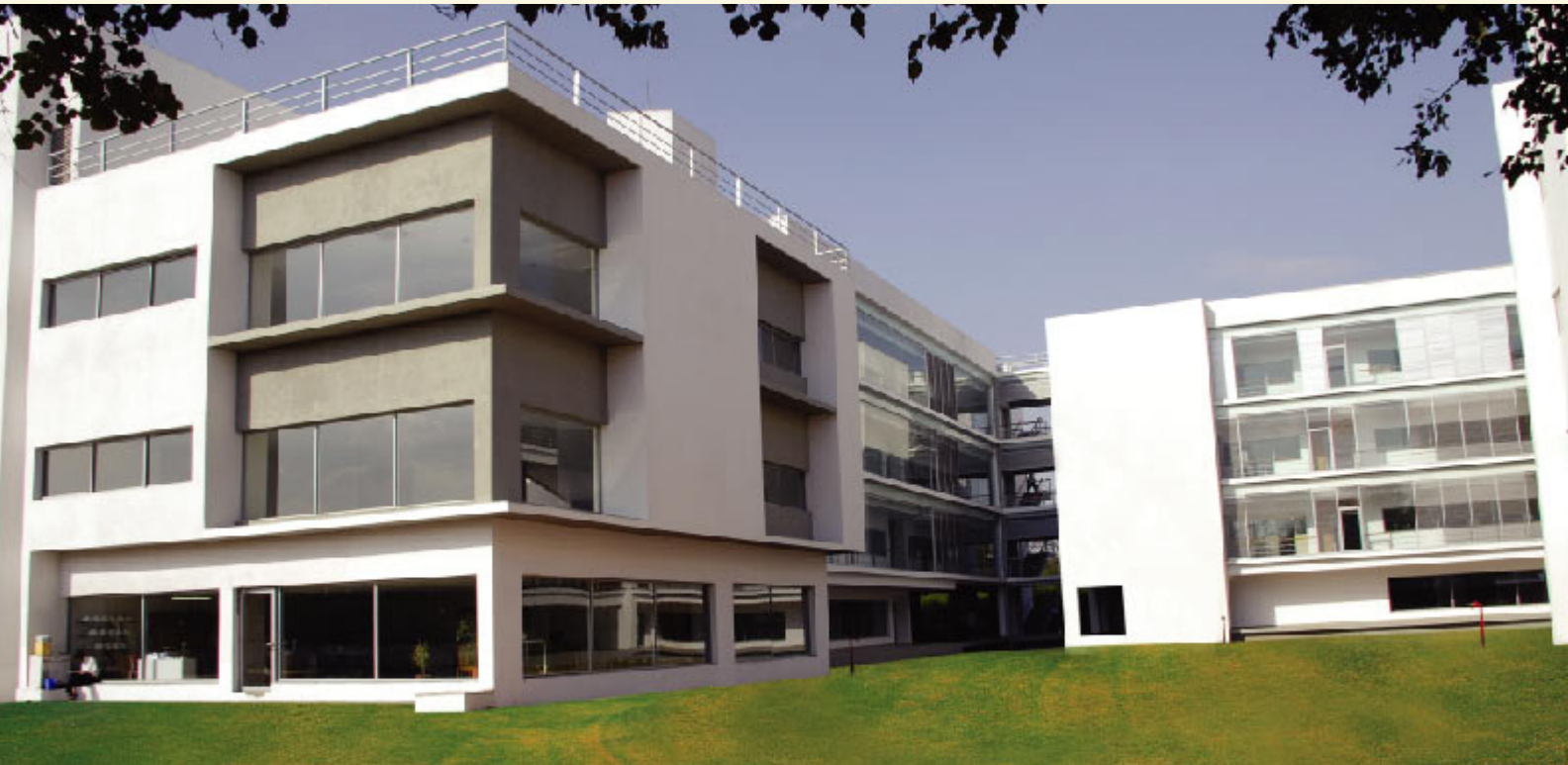
New laboratories at R&D facility, Bhat
