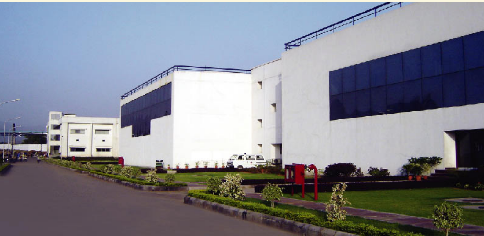
Manufacturing facility, Baddi, Himachal Pradesh
